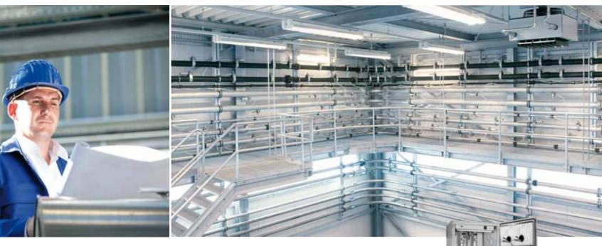
For the gentle conveying of sensitive bulk material such as carbon black and silica, the lowest possible conveying velocity is essential. To ensure a dust-free environment in and around the plant, the powdery raw material has to be conveyed pneumatically in closed systems.
