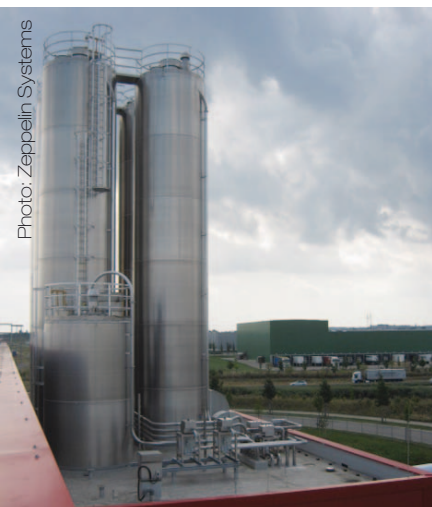
Left photo: The external silos are installed on the roof of the raw material storage which involved specific structural requirements. Middle photo: The individual silos of the main components are built in such a way that they do not take up any space in building. Right photo: Ingredients are first weighed and then fed into the spiral mixer.
