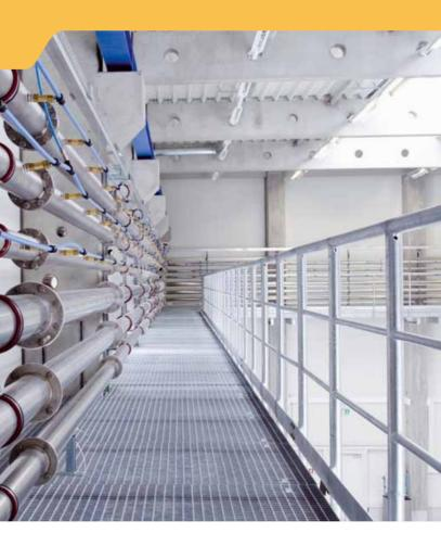
» Secondary air conveying DN 65 – 125/80 – 320 m » Bullet conveying pressure-/vacuum DN 65 – 110/80 – 240 m » Dilute phase conveying DN 65 – 110/80 – 240 m pressure-/vacuum
